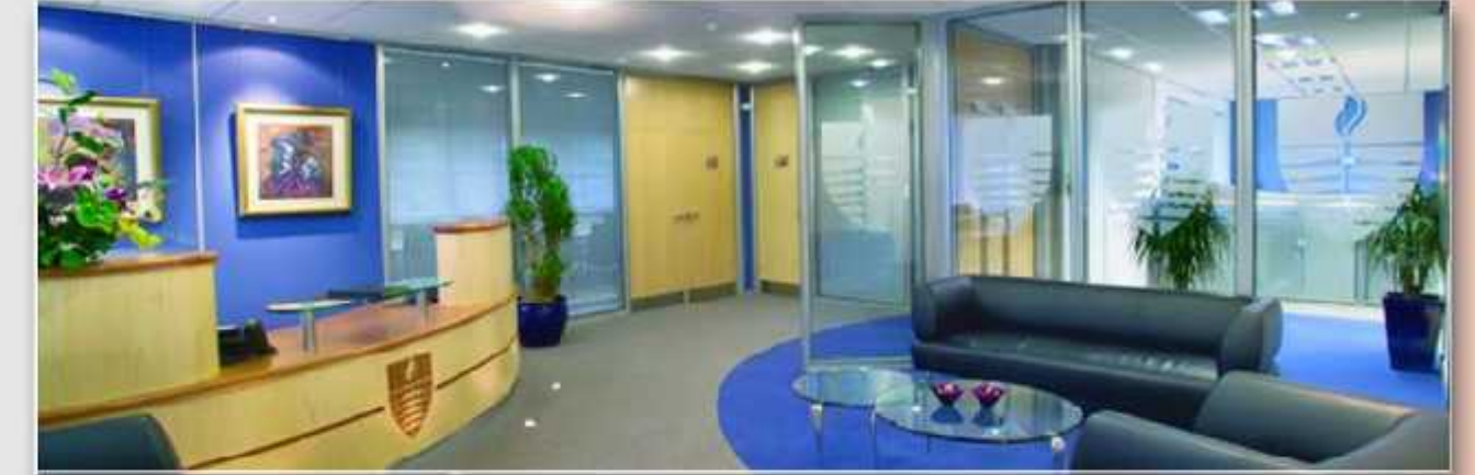
Reception with Demountable Partitions
