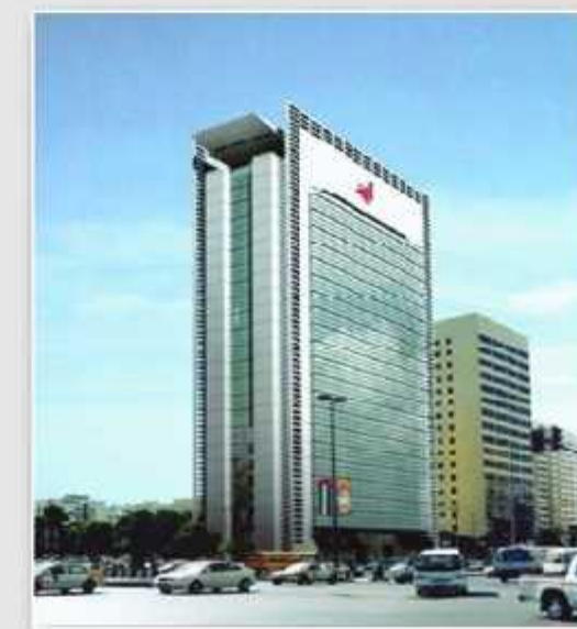
Abu Dhabi Commercial Bank (ADCB) Head Quarters
